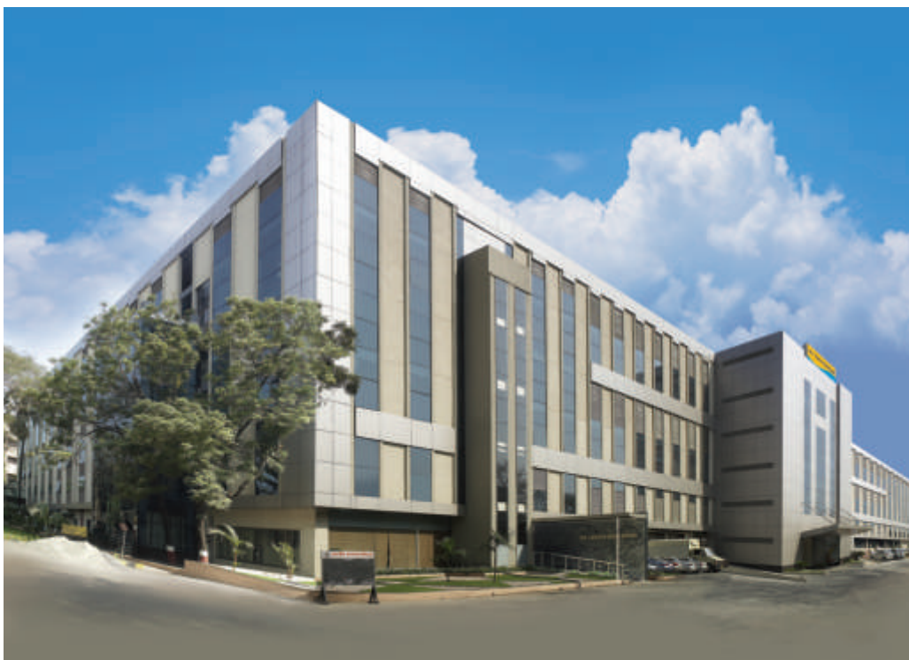
Switchgear Factory, Mumbai
